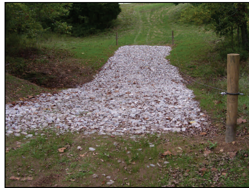
Stream crossing installed in Silver Creek Watershed
